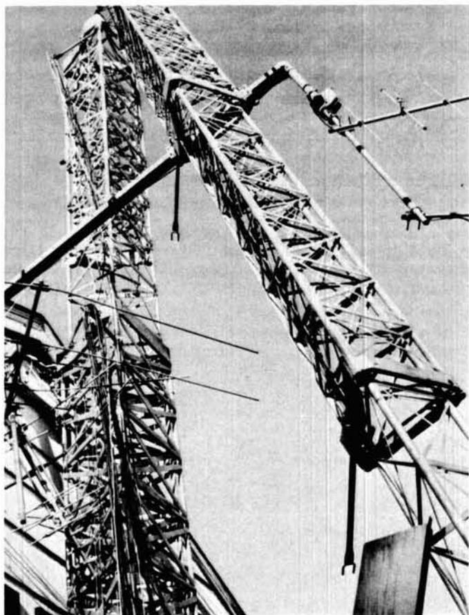
fig. 6. The winter storms hit, and the tower fractured at mid-joint. Luckily, no one was injured when all of this metal tumbled down from the sky. Is your antenna designed to stay up?
